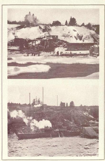
HE months of February and March were very cold and stormy. Snow was on the ground and at times to the depth of three feet. Consequently very little progress was made excepting in the building of cofferdams, which were easily handled through the ice, and in the erection of necessary buildings for storage and for the convenience of laborers. The construction plant was also received and set up and by the first of April the ice had gone out of the river and the site had been practically cleared.
